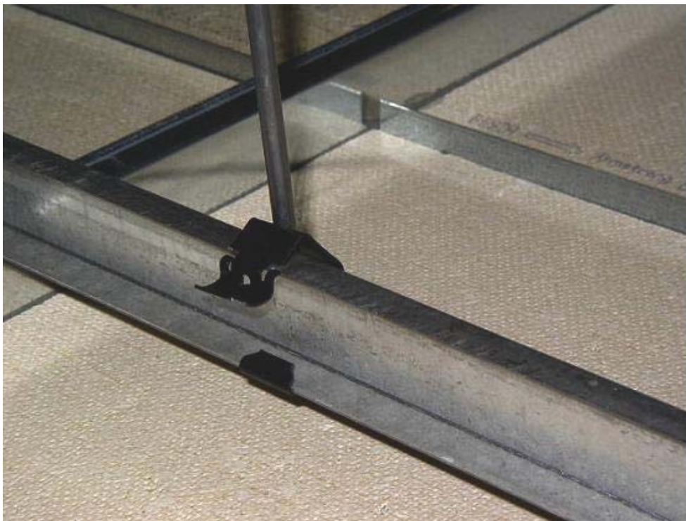
Figure 2–17. Bottom CADDY fastener in suspension system 1.
